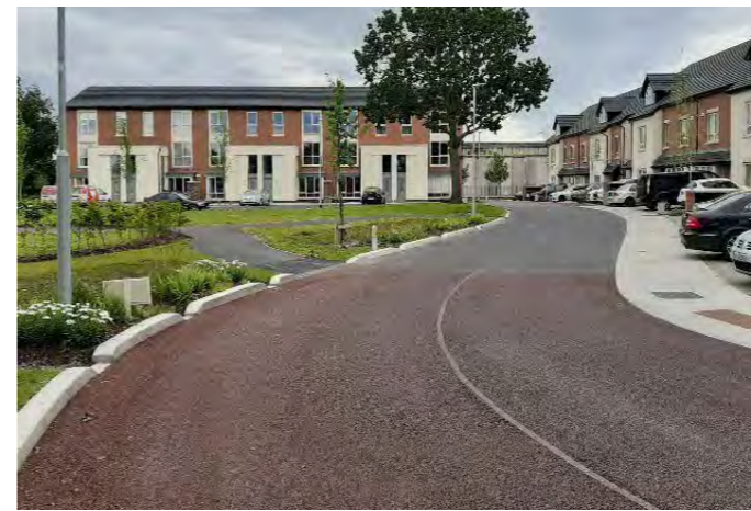
Coloured Asphalt Surfaces - to paths and shared surface roads, (see engineers drawings for type).
