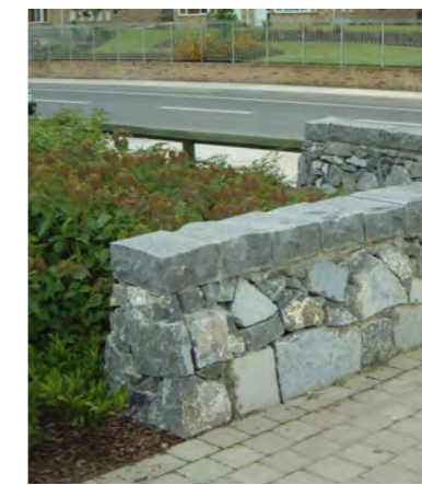
Reconstituted stone Concrete block and natural stone walls using local vernacular style, as informal seating areas and to create terraces.
