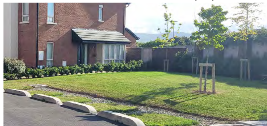
Breaks in the kerb allow surface overflow into the filter strip
