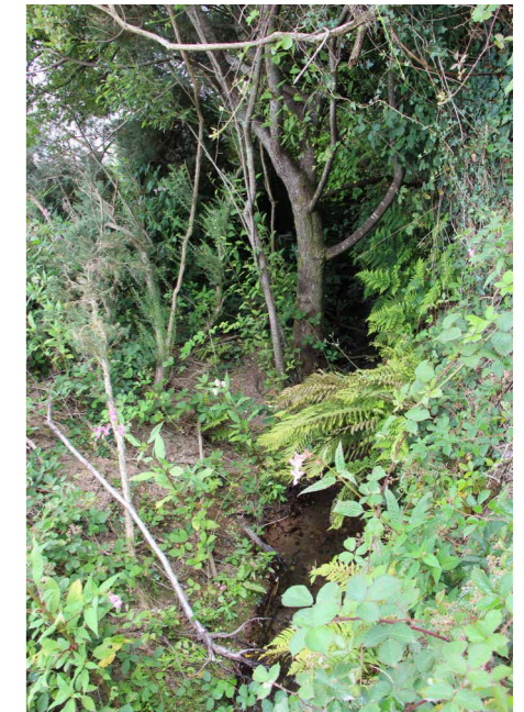
Existing central drain relatively dry and overgrown by vegetation
