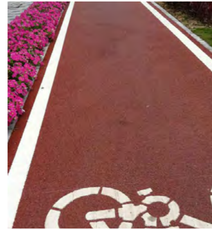
Coloured Asphalt Surfaces - to paths and shared surface roads, (see engineers drawings for type).
